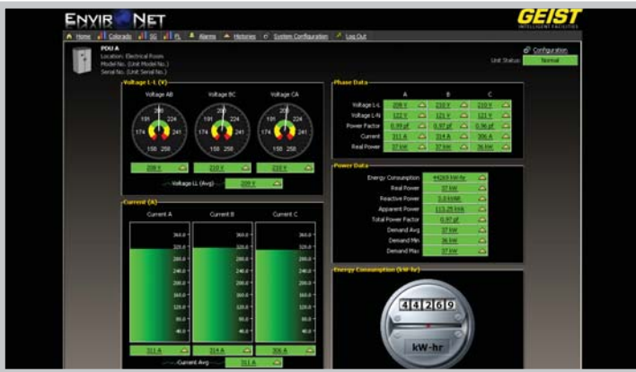
REMOTE POWER PANEL VIEW
